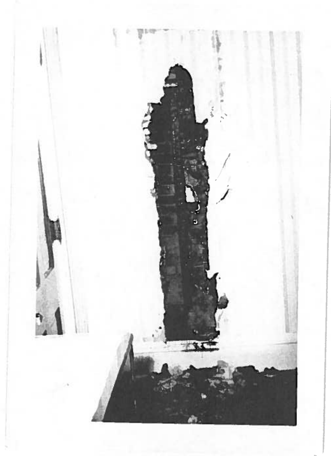
West wall of the bedroom behind the fire place. Fire traveled up the inside of the wall into the attic.
