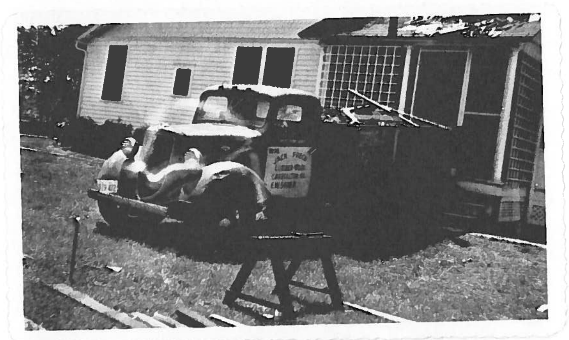
East side of the house during the repair process after the fire. Shows fire debris from the attic being load from above the screened in porch south of the rear door of the home. Truck belongs to Wm. Jack Frech Lumber-Wood, Carrollton, Illinois
